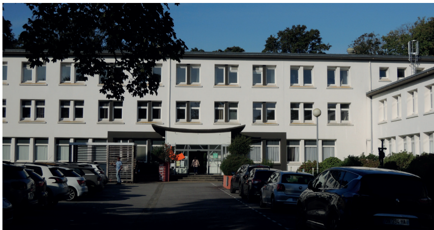
Centre de formation continue AREP 29 (Keraudren, Brest)
